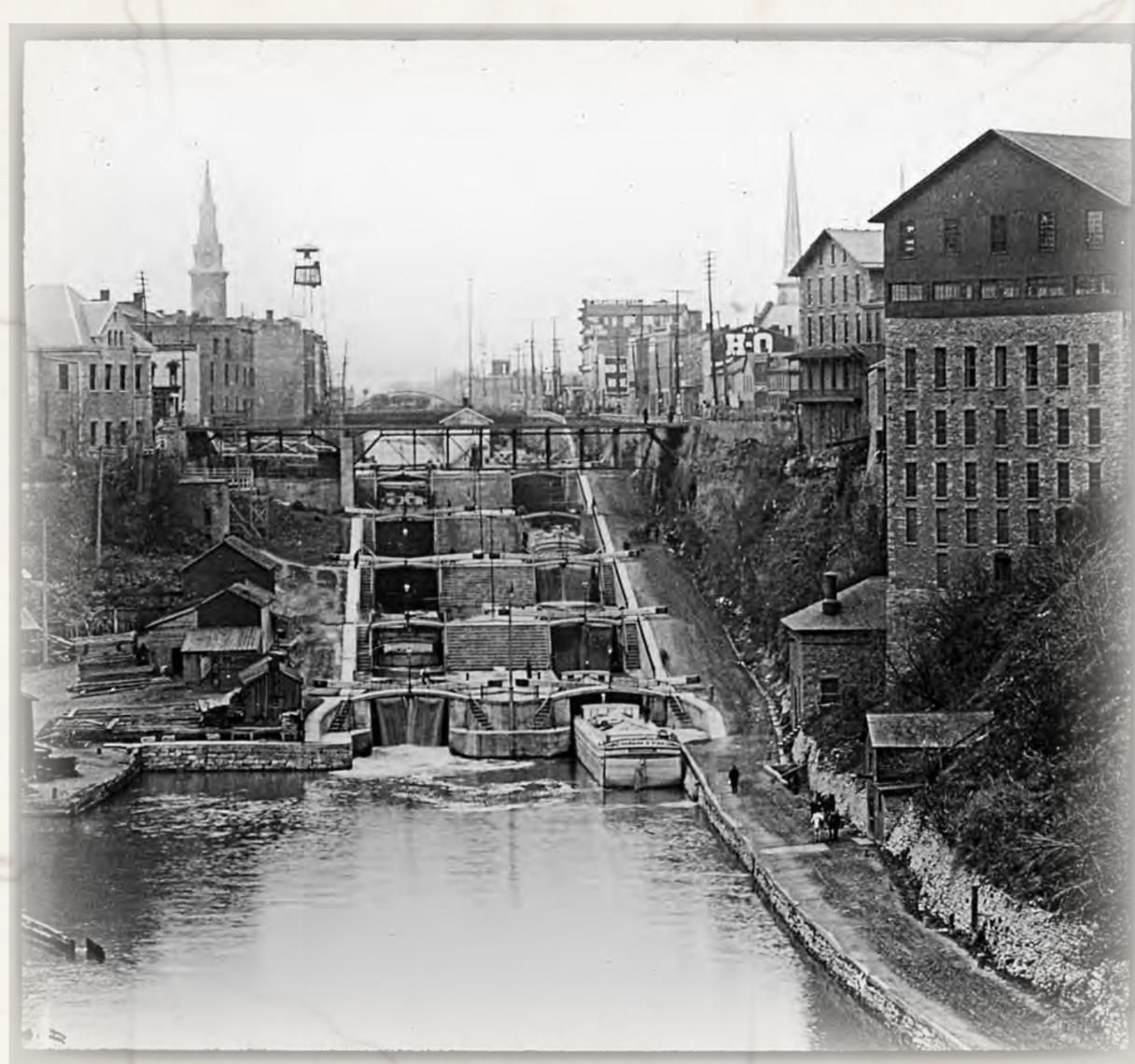
The most difficult engineering challenge was the Niagara escarpment at Lockport. It was essentially a 75 foot high wall of rock cliff and no lock had been designed that could handle that kind of lift. Nathan Roberts designed an ingenious "flight of five" locks to handle the lift in segments. The locks have undergone extensive renovations in recent years and are a popular tourist site.
